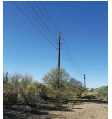
Typical 69kV double-circuit pole
