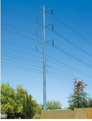
Typical double circuit 230kV power pole with double circuit 69kV underbuild
