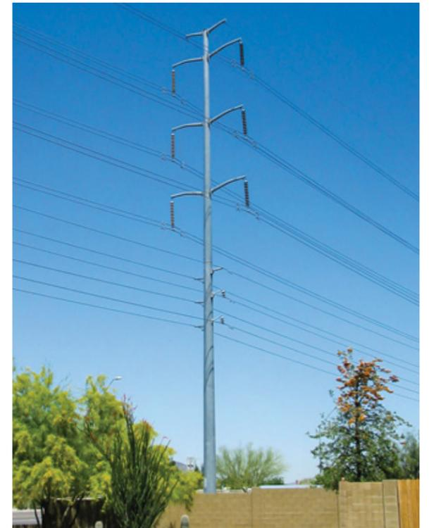
Typical double circuit 230kV power pole with double circuit 69kV underbuild
