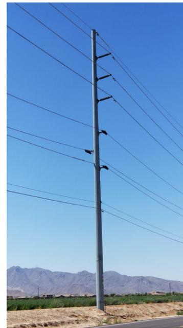
Single-circuit 69kV pole with 12kV underbuild
