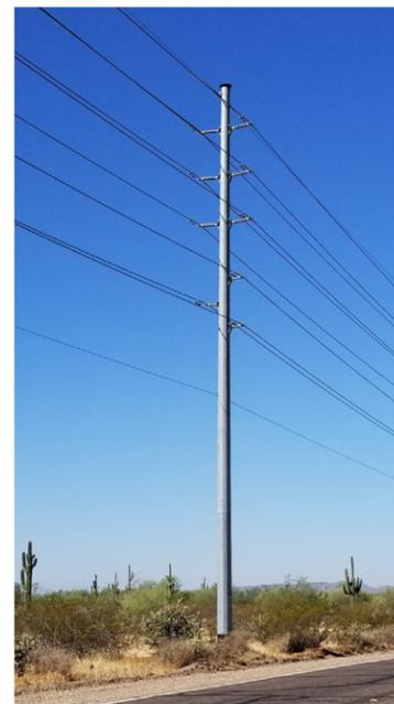
Double-circuit 69kV pole with 12kV underbuild
