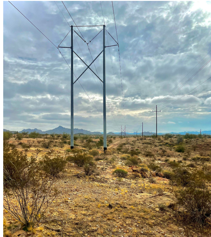
Typical H-frame structure
