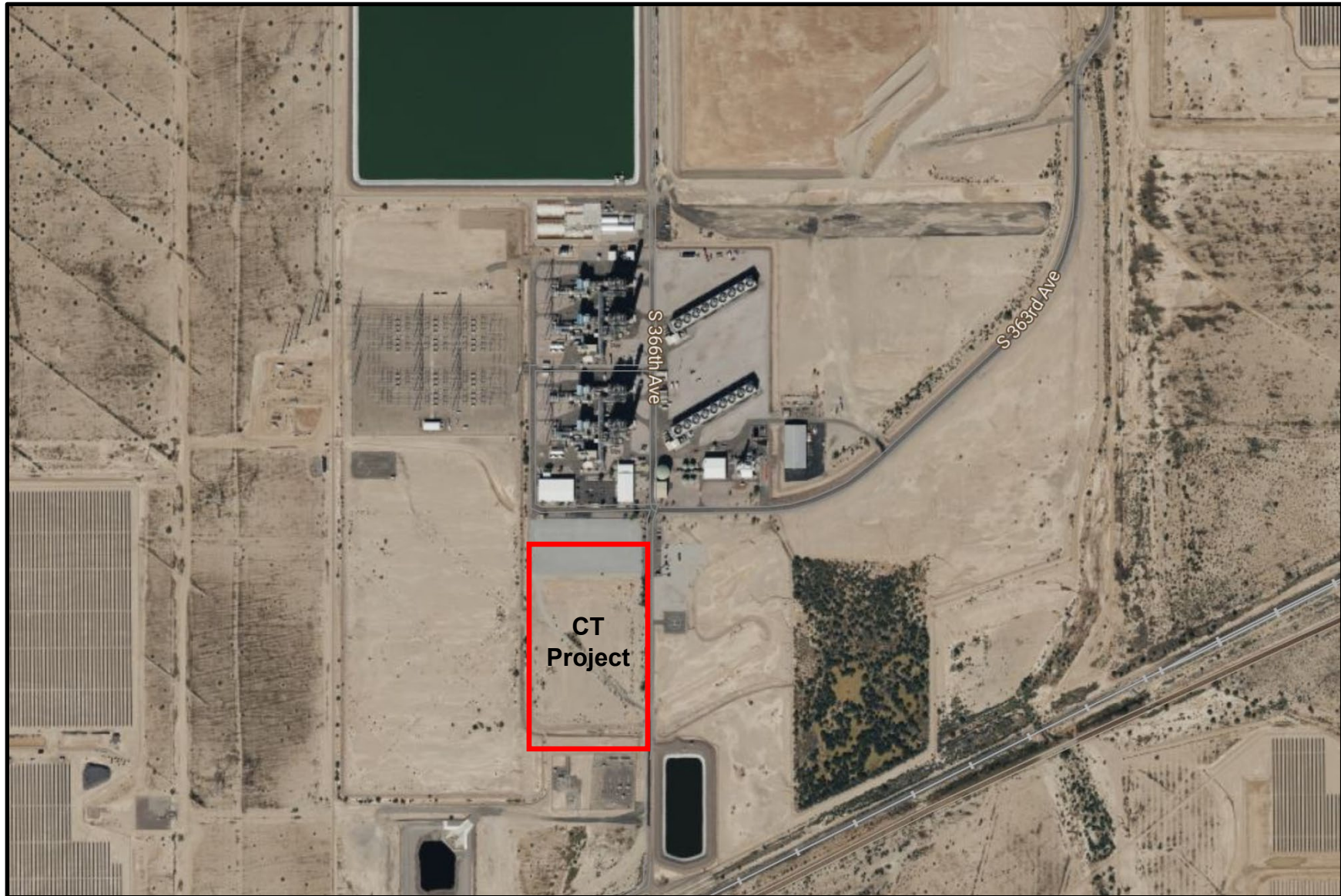
FIGURE 2-3. Redhawk Power Plant aerial image and location for the CT Expansion Project.
