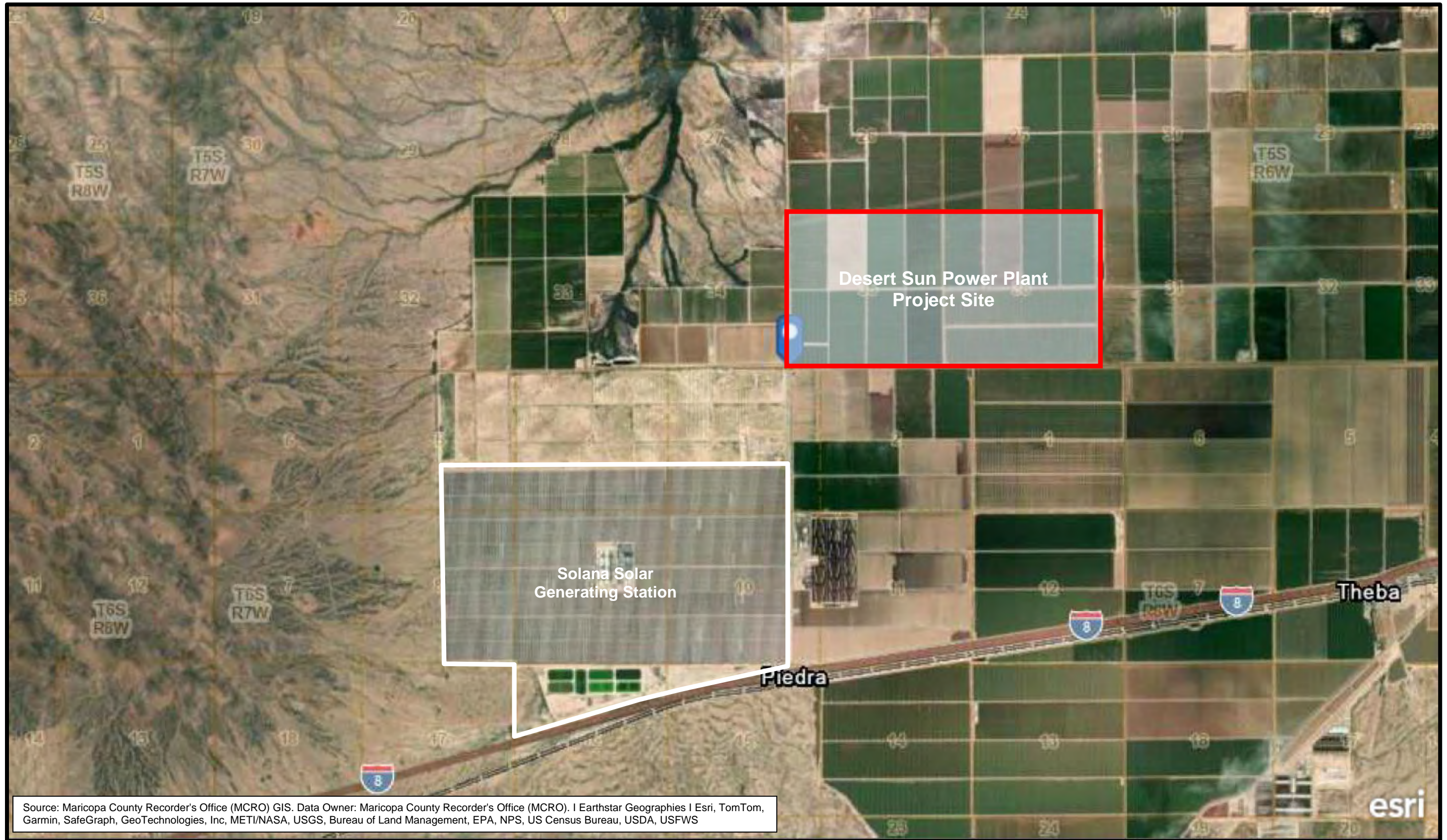
FIGURE 2-2. Aerial image of the location for the Desert Sun Power Plant.
