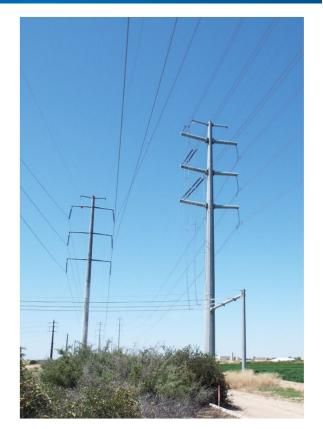
230kV Cut-In / 230kV Tangent (example photo)
