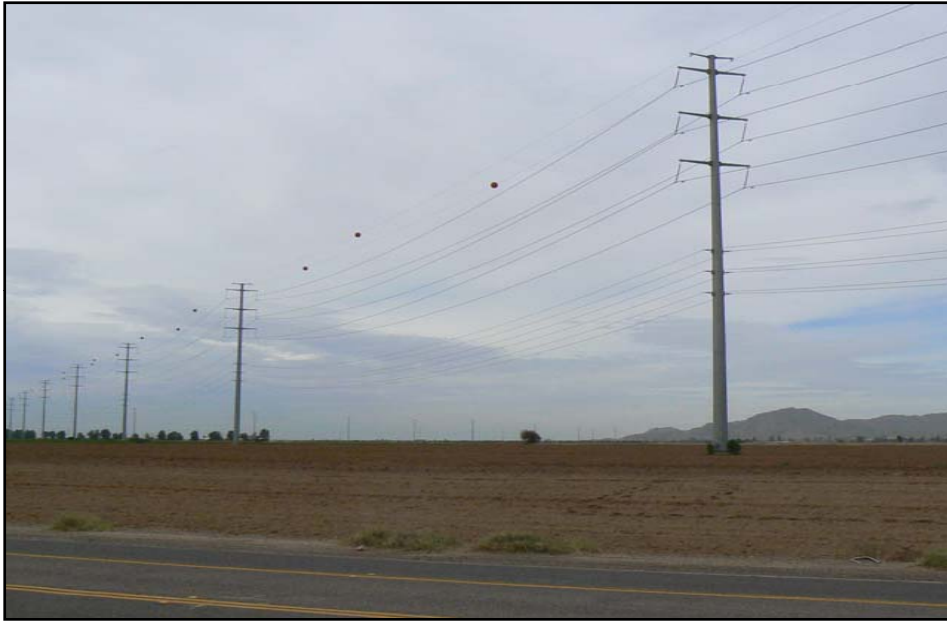
Typical Double-Circuit 230kV Transmission Structure with 69kV Underbuild
